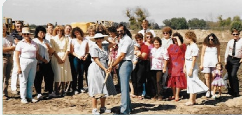
SJVC campus groundbreaking
